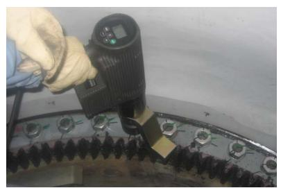
The Torque and Angle Capability of the Titan ATEip 2200-P16 PLUS provides quick work of the T-bolts (blade to blade bearing) to 413 ft/lbs <u>plus 120 degrees rotation</u>. On this turbine there are 60 bolts per blade on the inside of the nose cone.
